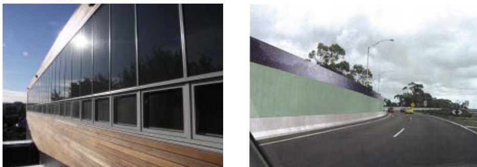
Figure 3 Left: the largest vertical north-facing BIPV façade in Australia, covering 200m 2 , commissioned in 2006 at Ballarat University (Going Solar and McIldowie Partners Architect); and (right) the pioneer use of PV panels to create a noise barrier wall at Tullamarine Airport (Going Solar, Melbourne). (Photo credit: www.goingsolar.com )
