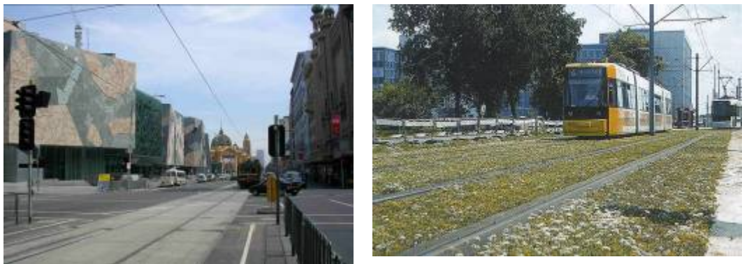
Figure 6 Green potential Left - tram lines in Flinders St, Melbourne (Photo credit: www-personal.umich.edu ) Right - tram lines in a European City with sedum vegetation mats laid as groundcover for amenity and water retention purposes.
