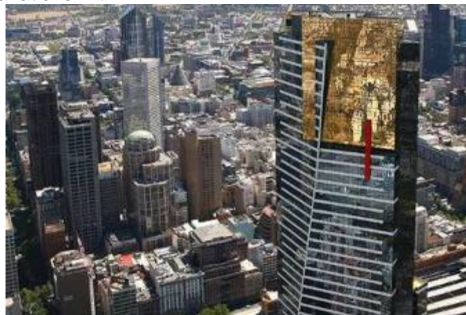
Figure 1 Endless possibilities: Melbourne’s facades could shape up for productive technologies. Solar panels might replace glazing, building might be retrofitted to capture water and grow plants. (Photo credits: Craig Abraham, Plain Jane Creations.)
